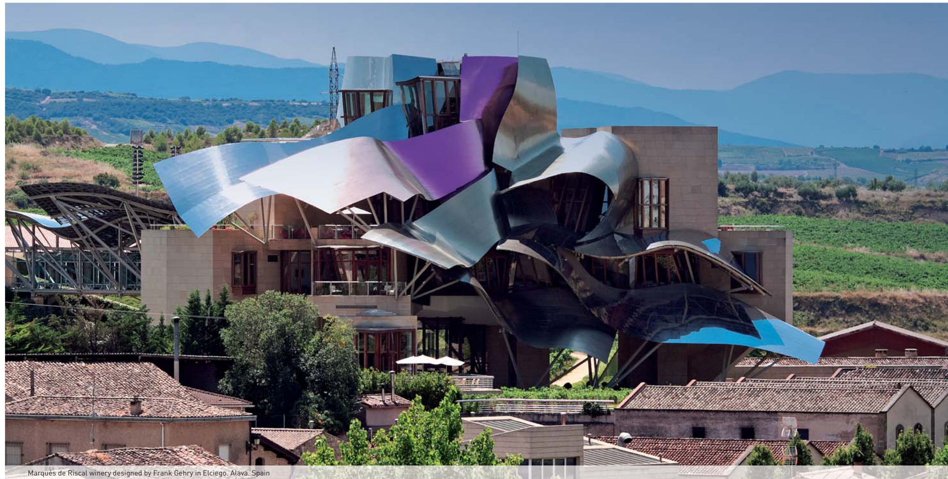
Marqués de Riscal winery designed by Frank Gehry in Elciego, Alava, Spain
