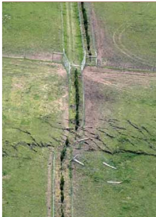
Figure 5: Example of farm fences displaced by surface rupture of the Greendale fault during the 4 September 2010 Earthquake. (Photo: Nicola Litchfield, GNS Science).
