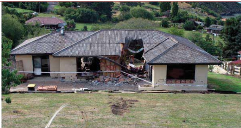
Figure 11: Example of boulder impact on house in the hillside suburbs (note the bounce mark in the foreground) (up), and cliff collapse threatening houses and occupants at both the top and base of the cliff (down).
