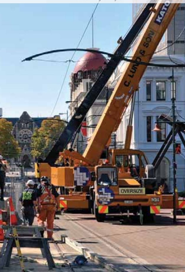
Workers stabilizing buildings at Worcester street, Christchurch
