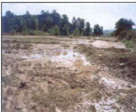
Rain damage to channel construction
