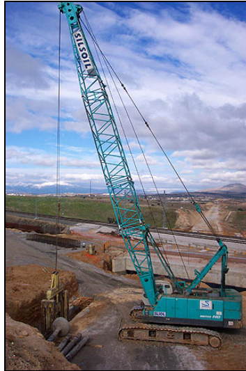
Diaphragm wall construction
