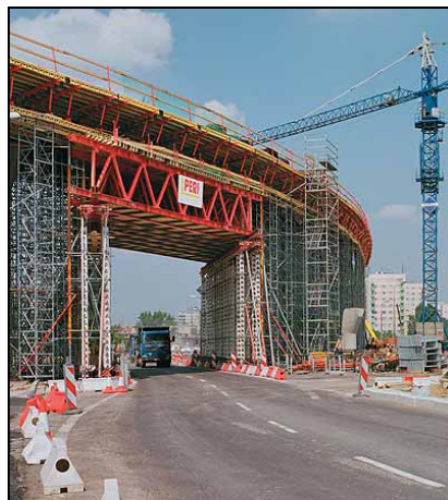
Falsework assembly. Crossroads in Czermiakowska, Warsaw, Poland
