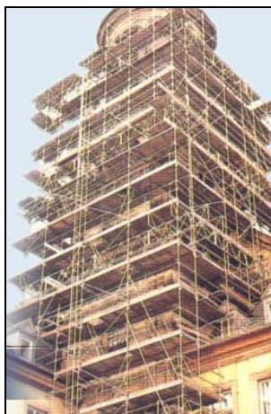
Scaffolding at building construction
