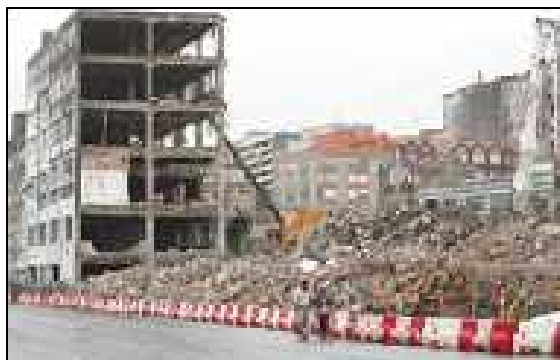
Debris after demolition
