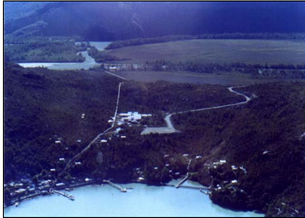
Construction site environment
