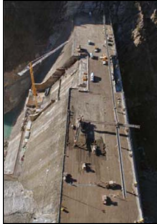
Ralco dam construction (Chile)
