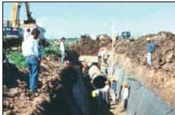
Accumulation of material near the trench
