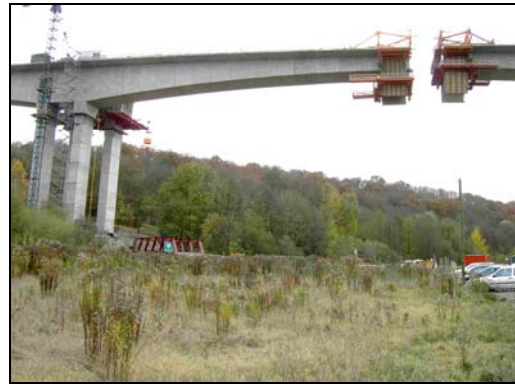
Cantilever bridge construction from piers
