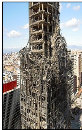
Windsor Tower (Madrid) after the fire
