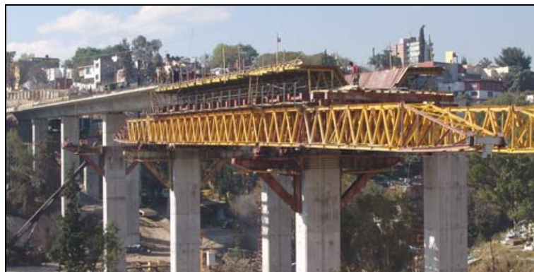
Sliding structure at Tarango bridge (Mexico)
