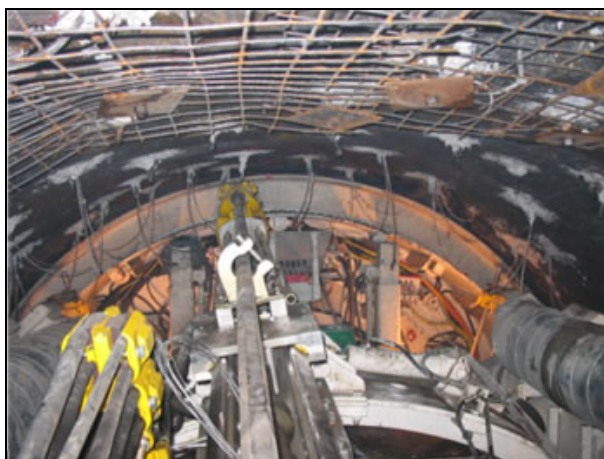
Underground excavation crown. Jointed ground
