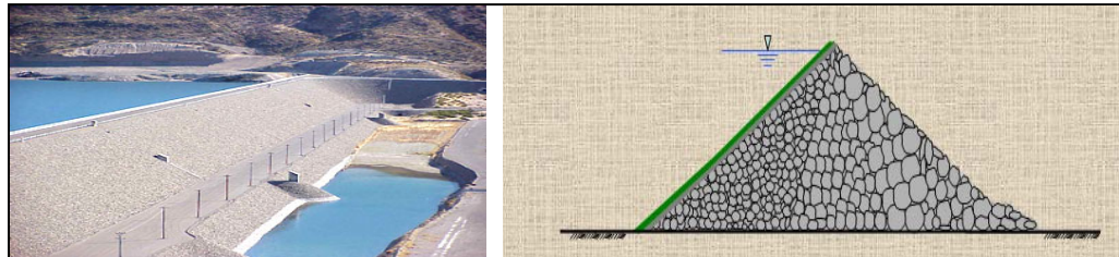
Heterogeneous embankment dam with impervious screen
