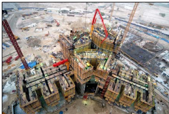
Concrete structure formwork
