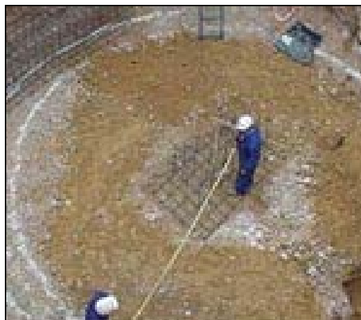
Setting out of works
