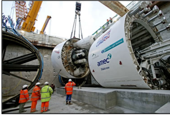
TBM (Tunnel Boring Machine)
