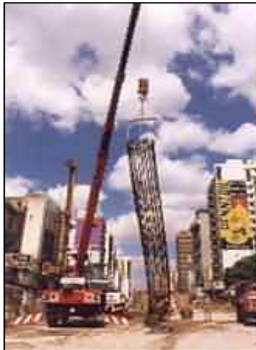
Insertion of pile frame
