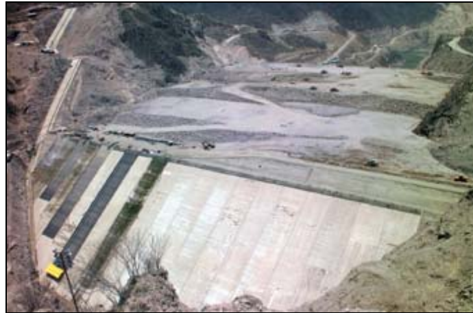
Execution of asphalt layer at Ralco dam
