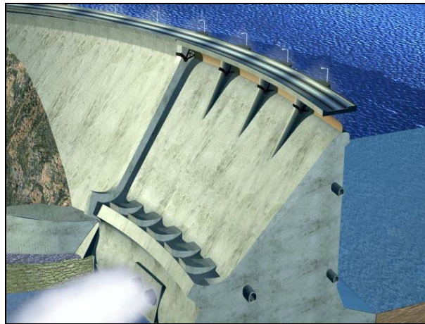
Double curvature dam
