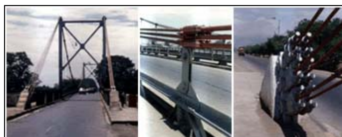
Suspension bridge. Detail of anchorage blocks
