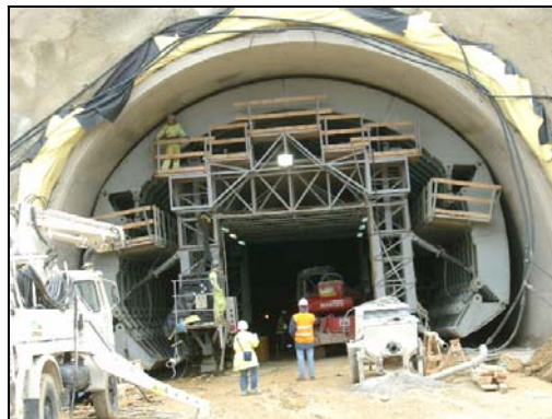
Dowells assembly in tunnel construction
